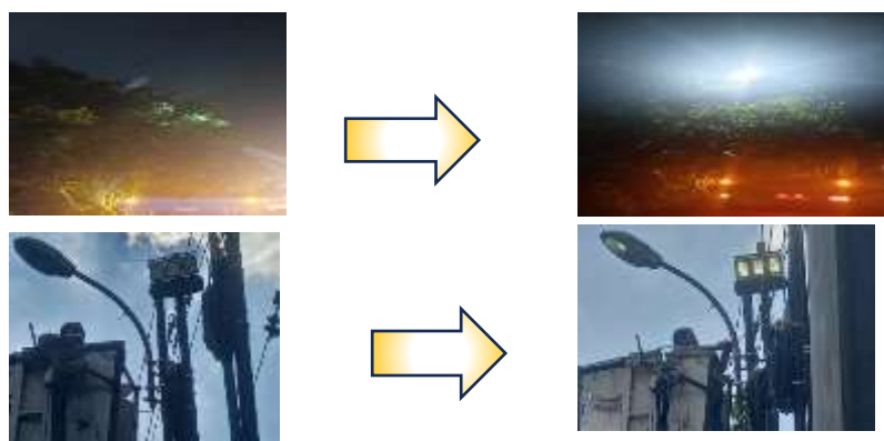
Figure 2. Some PJU Points Outage and Repair
